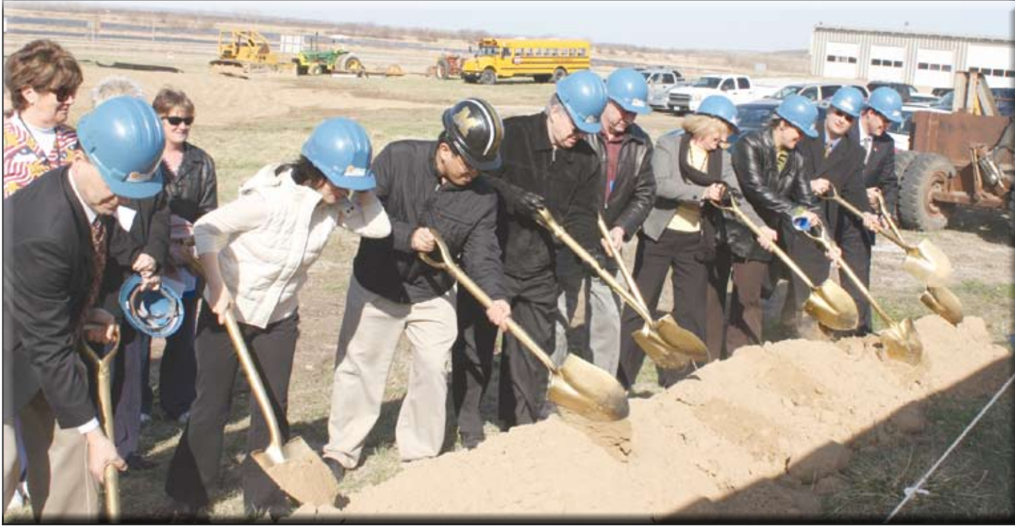
Northwest Health Services- Broke ground for a new building on Monday, March 30. Board members and others directly involved in the project were on hand with the traditional gold shovels to help get the project officially started.
