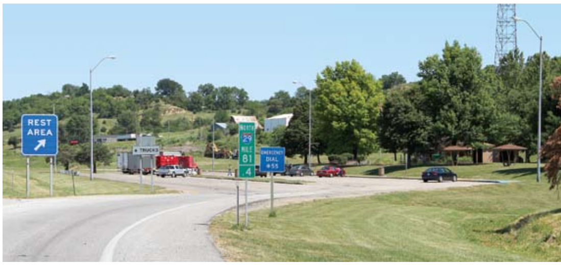
The northbound rest area on Interstate 29, just south of Mound City- Is scheduled to be demolished beginning on Monday, June 4. Both rest areas will be destroyed and paved for truck parking with only unimproved facilities located on both sides of the interstate.
