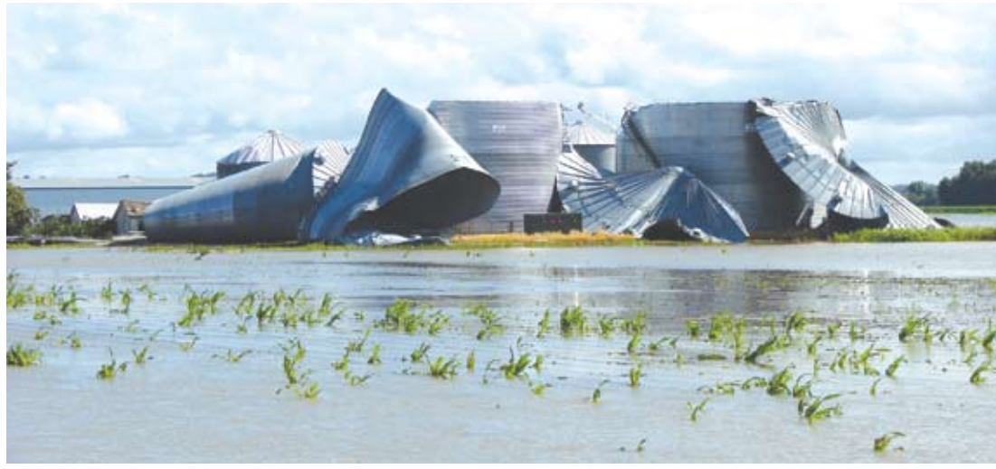
The remains of five grain bins- Are shown strewn along this high ridge at the home of Eddie Drewes, south of Craig, MO. The bins, which were empty and still dry despite being surrounded by floodwaters, were apparently destroyed by tornadic activity in the late night and early morning hours of Sunday and Monday, June 26 and 27. The roofs of two 50,000 bushel bins were torn off, and two 20,000 bushel bins were torn off their foundations and tossed into the 50,000 bushel bins. Skylights in the home at the same property were also sucked out and a large tree was ripped up and dropped onto a tractor.
