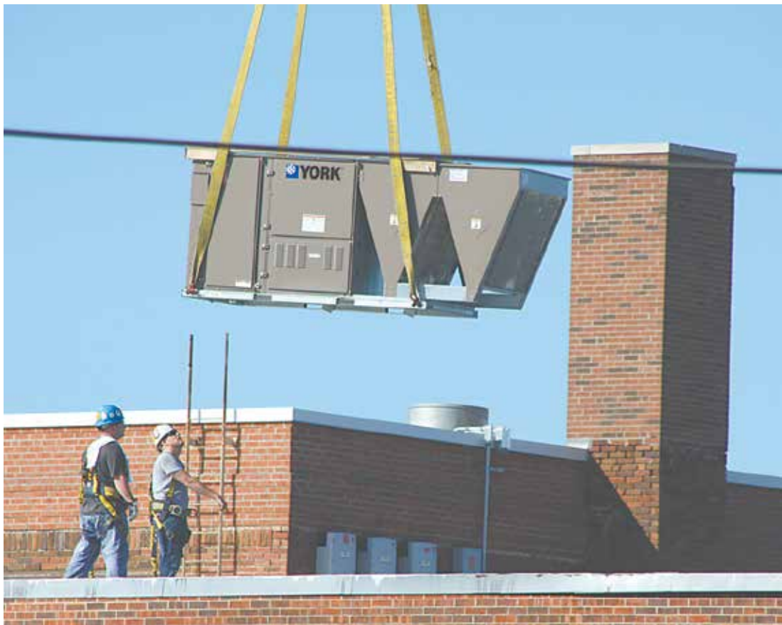
Employees from Brooner Construction and Crane - Guide one of the large air conditioning units onto the roof of the gymnasium at Mound City R-2. The patrons of the school district passed a bond last year that included the installation of new heating and cooling units throughout the school.
