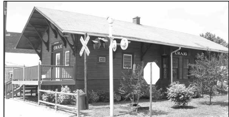
The old depot was moved from beside the railroad tracks and refurbished for use as City Hall.
